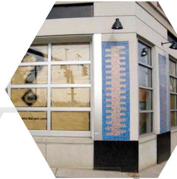
NATURAL STONE & GLASS MOSAIC INSTALLATION
